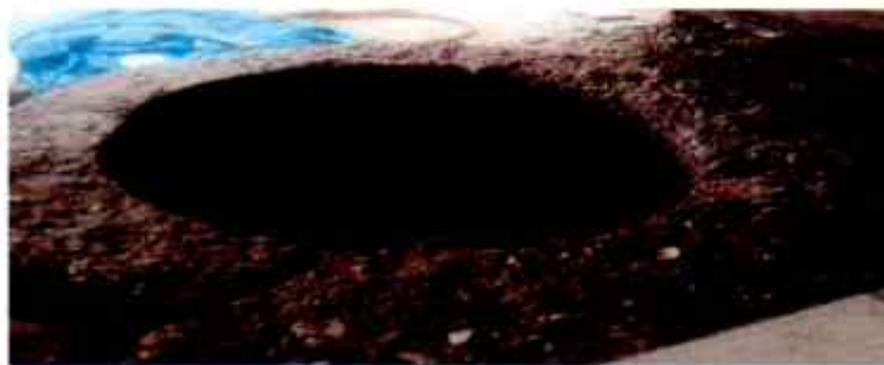
Fig 11:- Biogas Tank in Khaira College, Khaira
